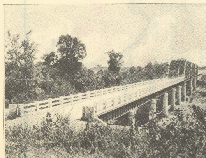
NEW BRIDGE OVER BOGGY RIVER—U. S. 70
