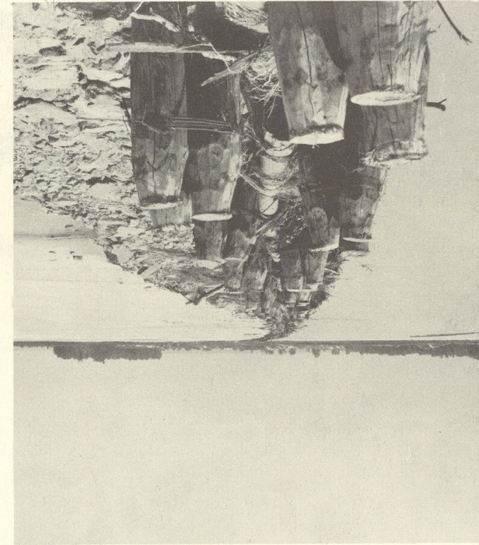
Pile dikes stabilize the future navigation channel of the Arkansas River near Fort Smith, Ark.
